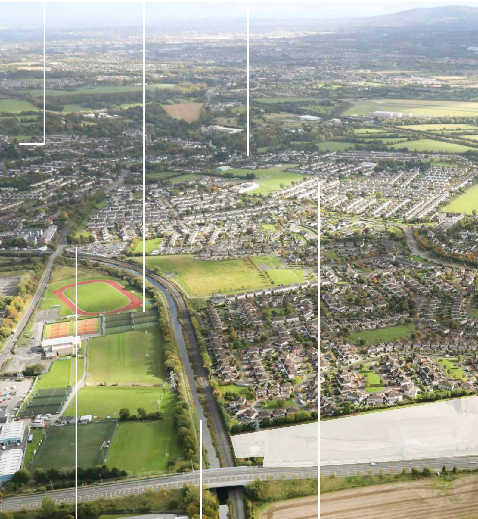
Louisa Bridge Train Station
