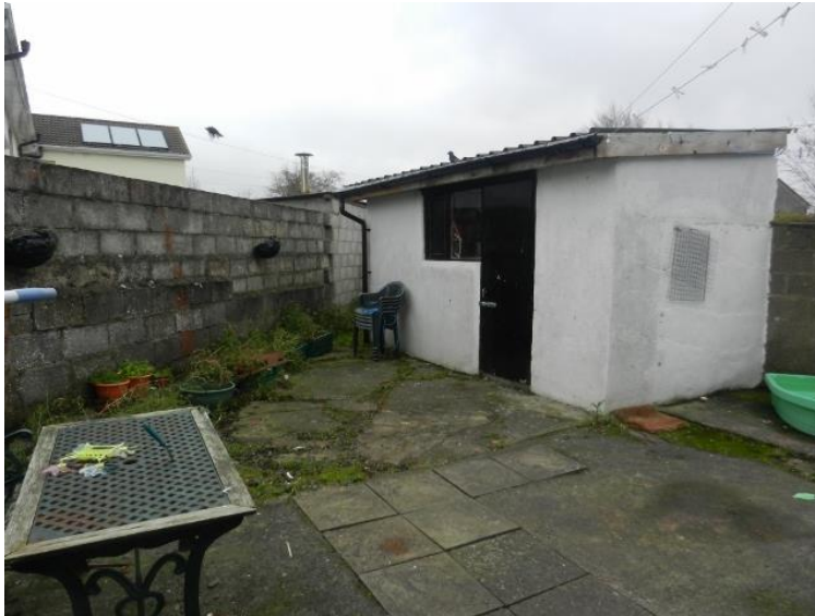
Walled in yard to rear with small block built shed.
