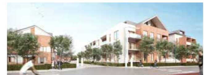
Station Road, Portmarnock
