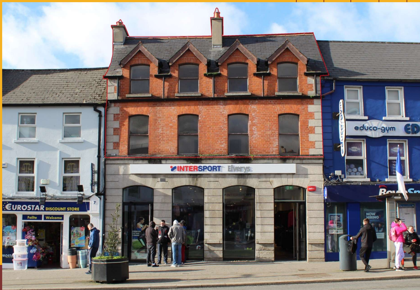
Westview House, Abbey Street Naas Co. Kildare
