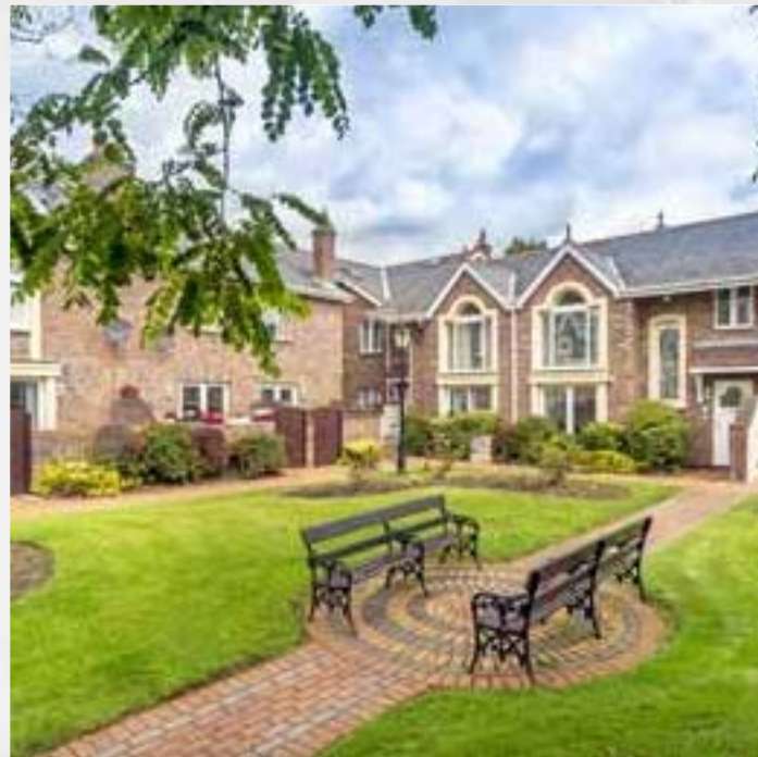
Simmons Court Square, Ballsbridge, Dublin 4.
