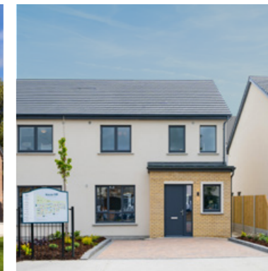
Ravens Mill Rolestown, Co. Dublin
