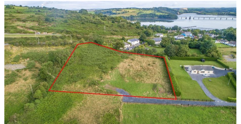
AERIAL VIEW SHOWING THE BARROW BRIDGE
