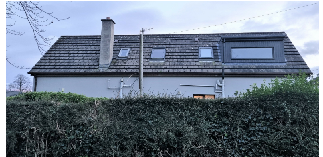
Existing House No 16 Castlefield Terrace A63W882
