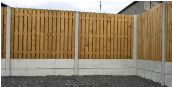
Concrete post & timber hit&miss fence
