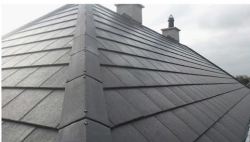
Sample - Roof Finish
