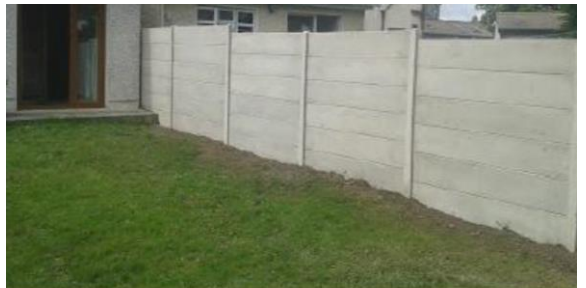
.8m concrete post & concrete panel
