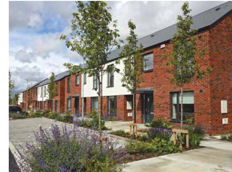
Stocking Vale North, Rathfarnham, Dublin 16 Construction of 175 family homes which were delivered to a very high specification.
