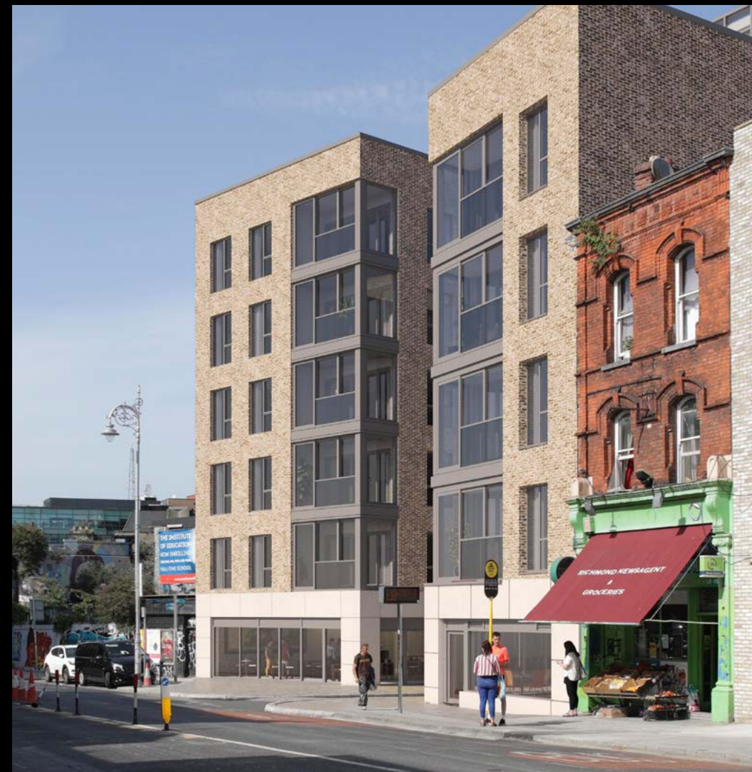
Richmond Street South Entrance Retail Units
