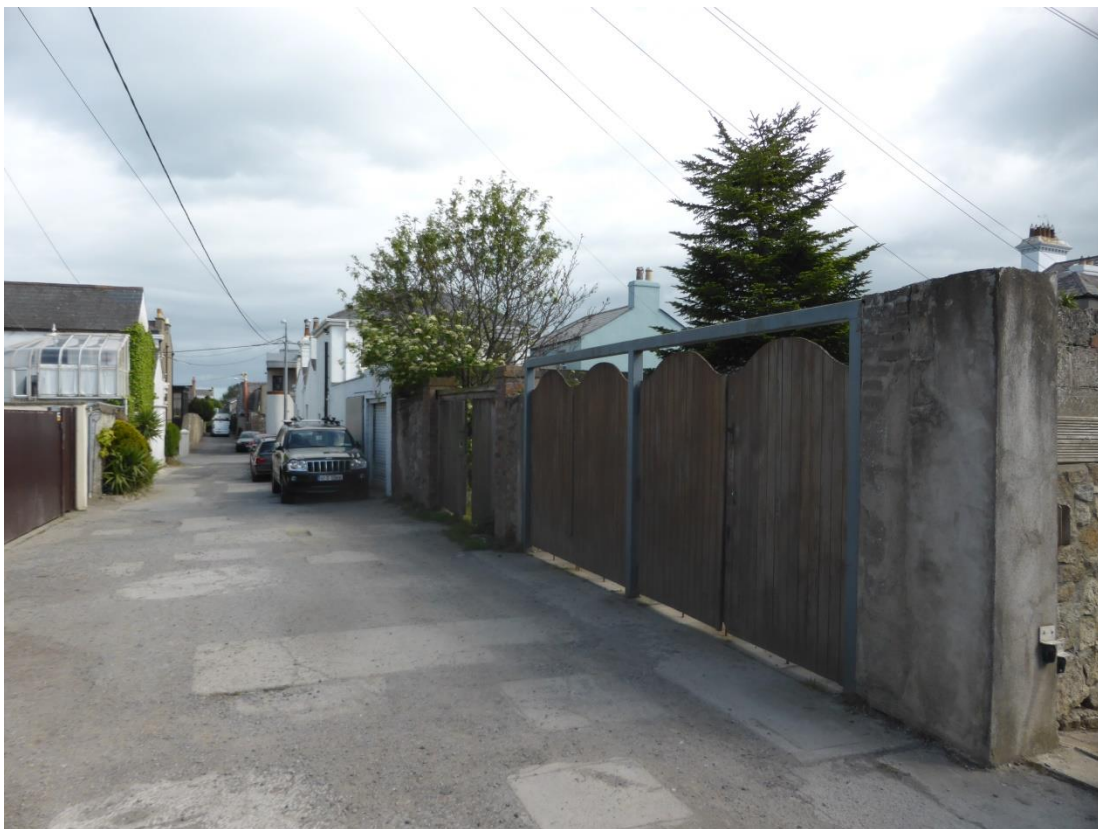
Existing Site Entrance – Boundary Wall & Gates
