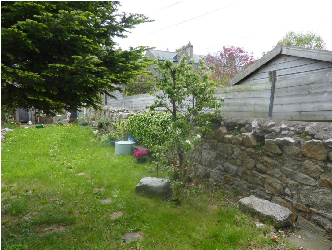
Existing Site Boundary Wall to be Retained
