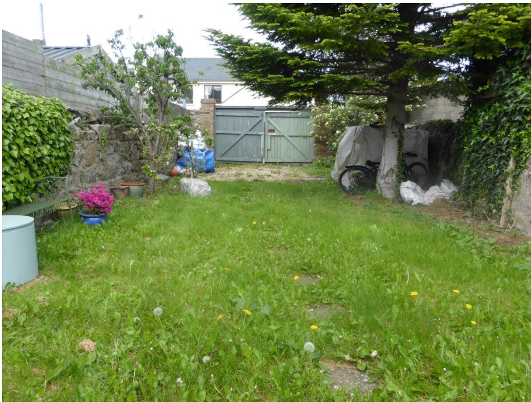
Existing Site Entrance – Boundary Wall & Gates
