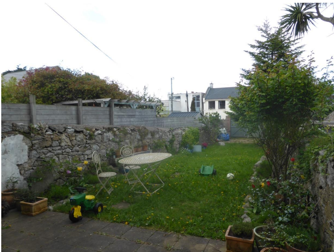
Existing Site Boundary Wall to be Retained
