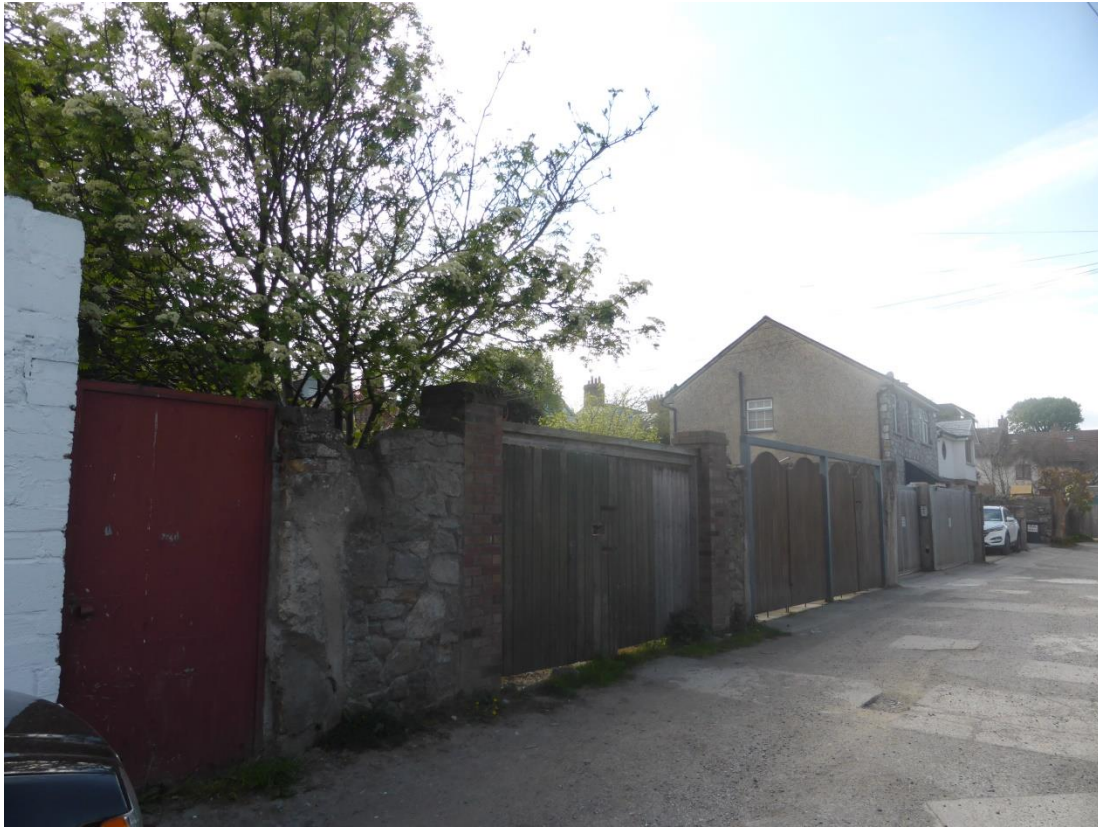
Existing Site Entrance – Boundary Wall & Gates
