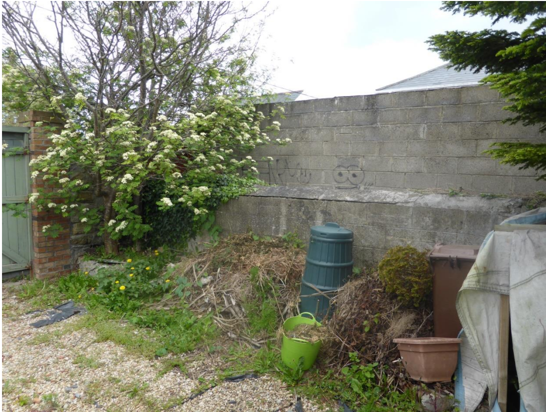
Existing Site Boundary Wall to be partially dismantled, Brickwork piers to be demolished.
