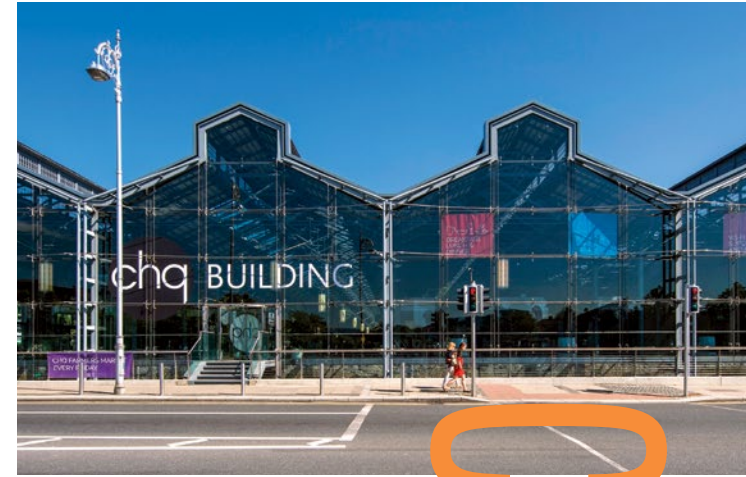
CHQ Dublin, 1 Custom House Quay
