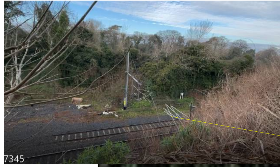
Escarpment to Railway - new fence
