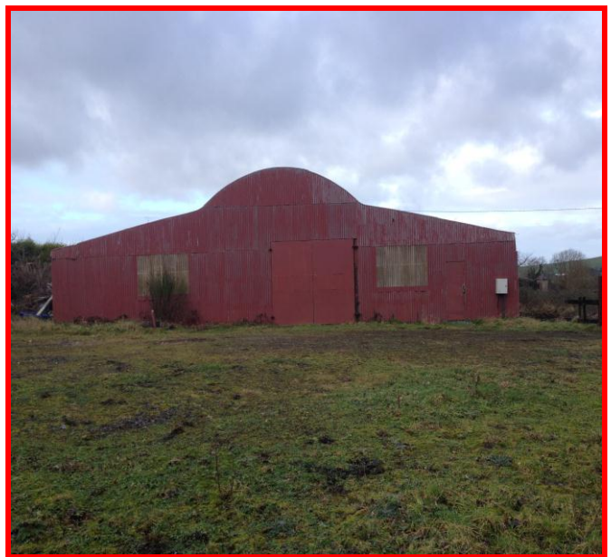
View of Shed
